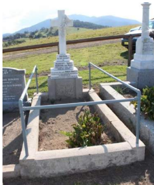
The monument was cleaned, and the surrounding handrail treated for rust and repainted.
