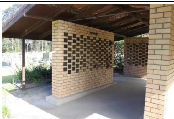
At Batemans Bay the niche wall has been integrated with a roofed structure.
