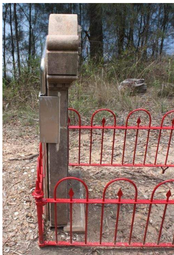
To support both upper and lower portions of the formerly broken headstone the steel plate has been embedded into the side of the stone. This minimises visibility from the front of the grave.
