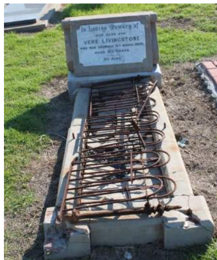
The monument was cleaned, broken pieces of the slab underpinned with loose aggregate and the rusted steel railings neatly arranged on the border.
