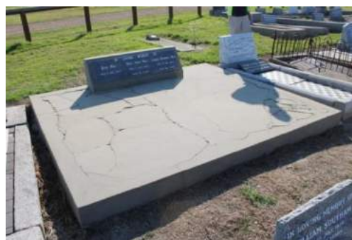
The slab was partially removed, underpinned and replaced as it had a significant cavity under it before the work was done.
