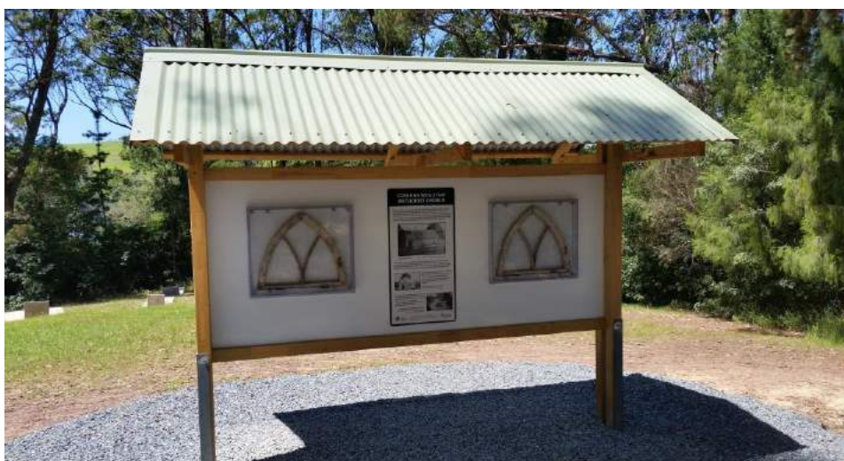
Corunna Cemetery interpretation shelter draws its inspiration and orientation from the former church that occupied the same site.
