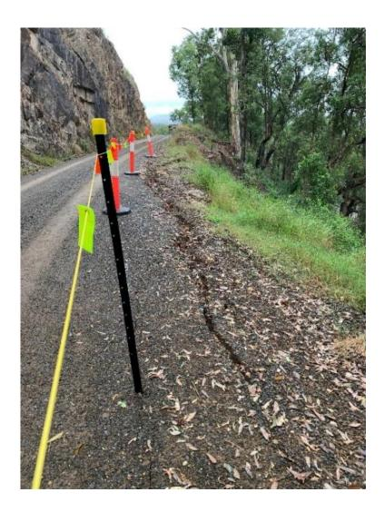
Tension cracking has developed in the downside embankment which requires more immediate stabilisation.
