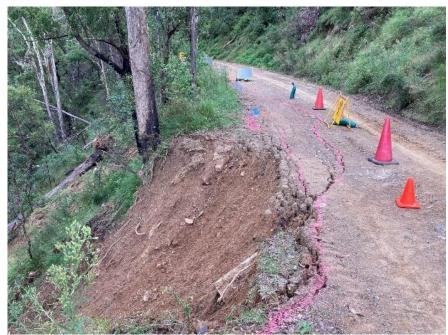
The proposed stabilisation works will enable the restoration of the road formation and provide ongoing embankment stability. Works will comprise Soil Nails, Shotcrete, Fibre Reinforced Concrete (Fibrecrete), Ground Anchors, Micropiles, Gabion Retaining Walls and other associated works are proposed to be implemented.
