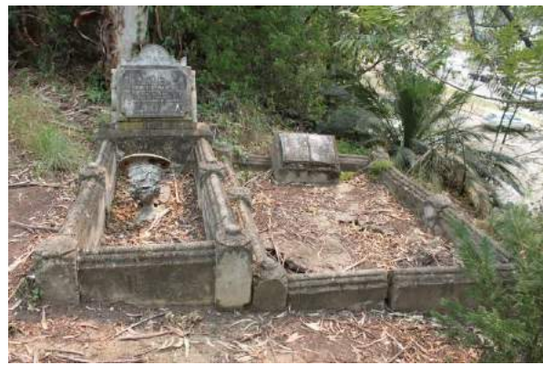
Plot is slipping towards excavated edge 2019
