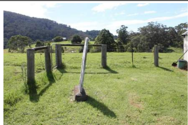
The stone could be carefully cleaned to reduce staining and the lettering checked and restored where missing. The stone leans forward and should be brought back to vertical.
