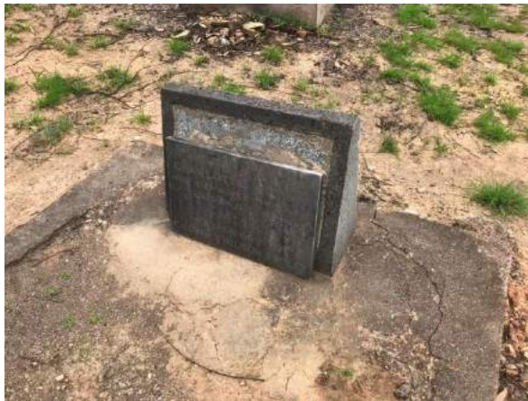
Heat has caused this plaque to detach from the headrest. March 2020
