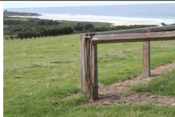
Termites have attacked the corner post as well as other posts and rails.
