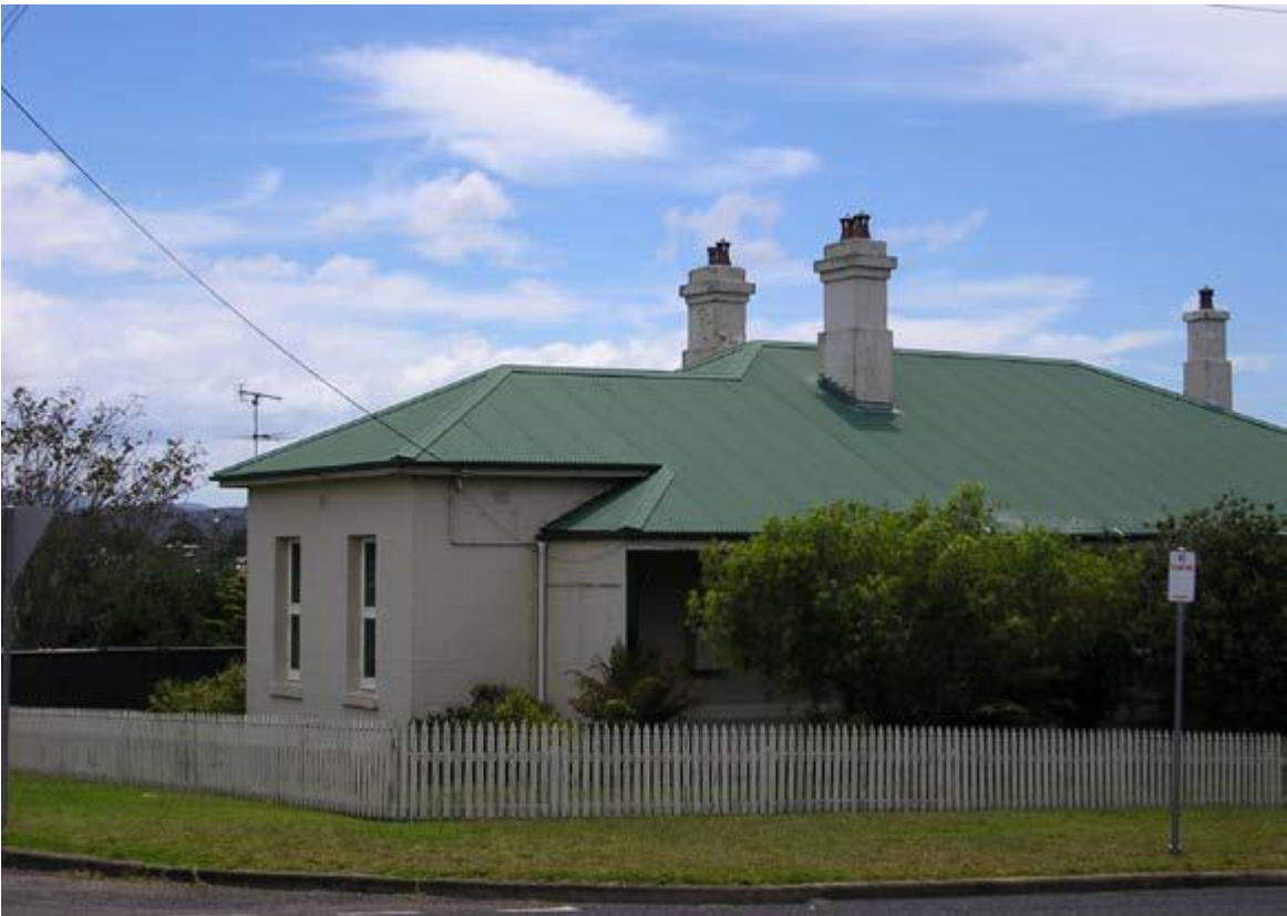
Early residential buildings Page Street- rendered construction.
