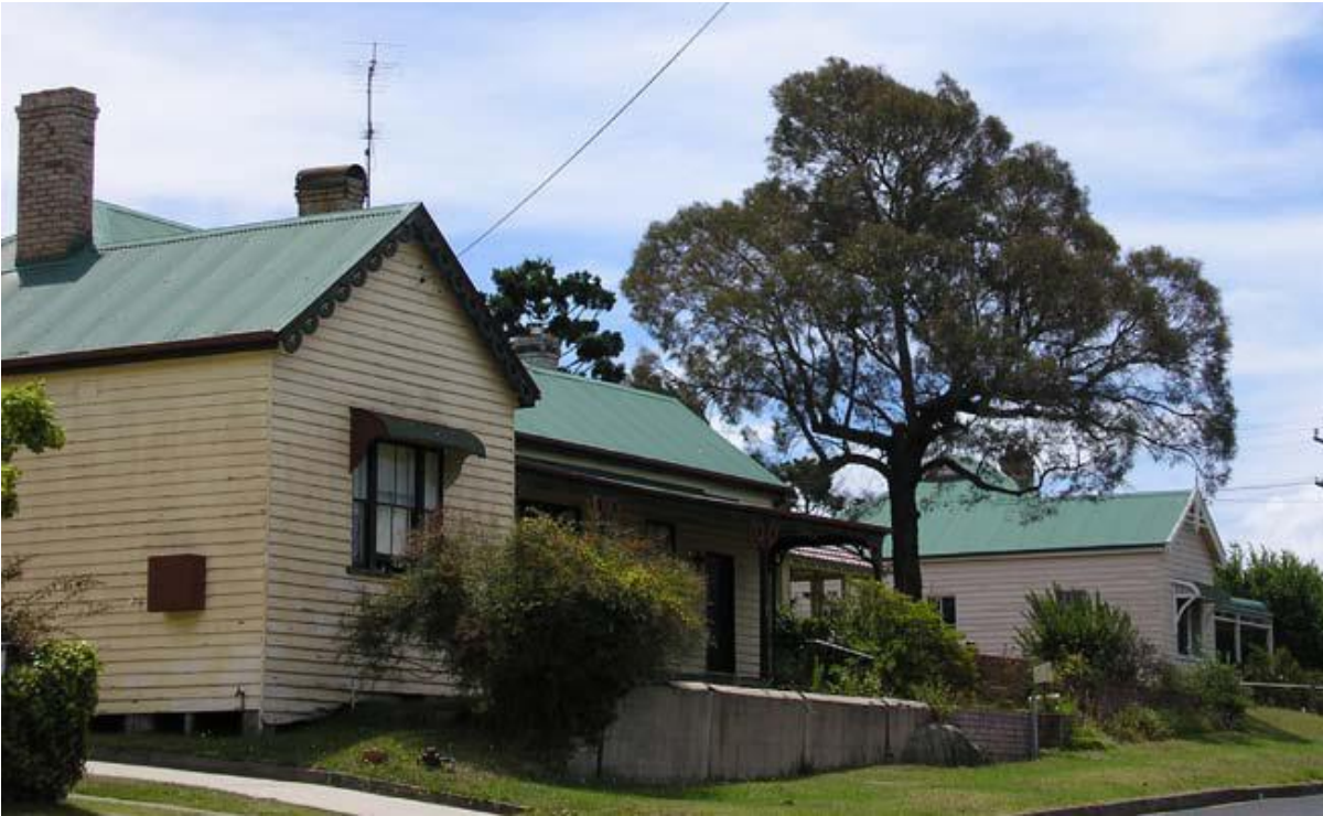
Photo: Early residential buildings Page Street. Building materials were weatherboards with corrugated iron roofs.
