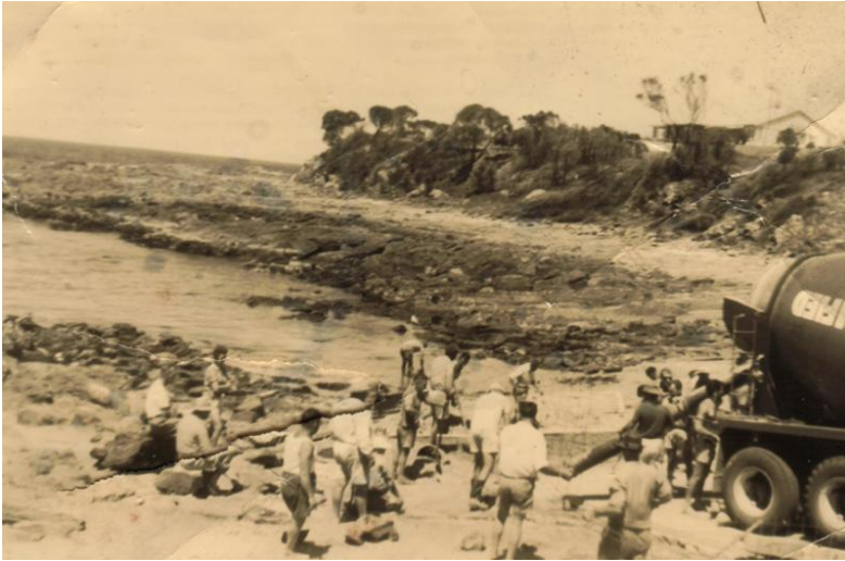
Locals pitch in to build a concrete boat ramp at Boat Harbour in 1961. Photo courtesy Wilding family.
