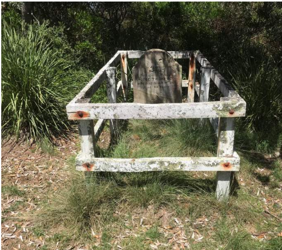
Photo showing active rust in the bolts and some timber splitting around the bolts. PG December 2017
