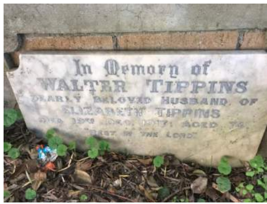
Walter Tippins. This memorial has dislodged from the wall. Also needs re-lettering.
