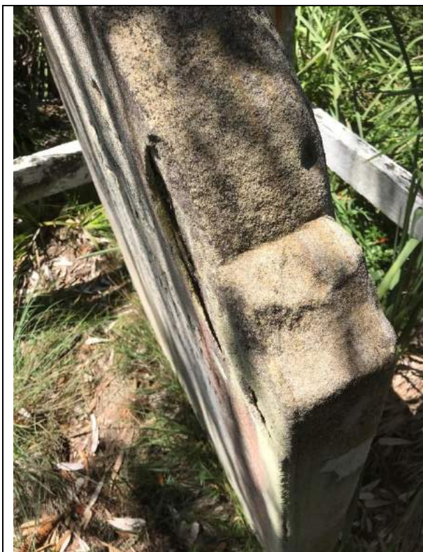
Delamination of upper right-hand corner of front face
