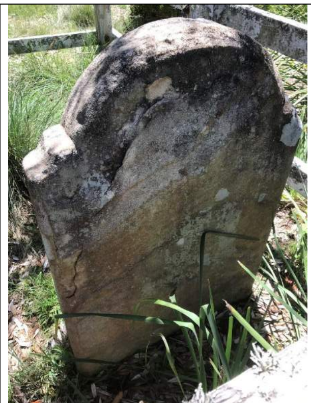
Delamination is also occurring on the rear face
