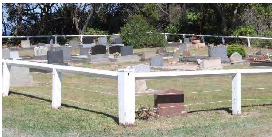
The painted post and rail fence at Narooma is an attractive and utilitarian style that clearly defines this section of the cemetery. A similar fence at Tilba district cemetery is being attacked by termites, which highlights the need to use durable timbers such as Australian hardwoods. Ironbark is an appropriate choice for historic cemeteries.
