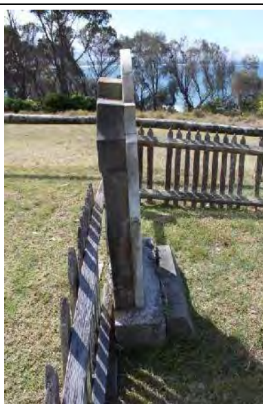
The thick concrete backing has been shaped to the stele's profile
