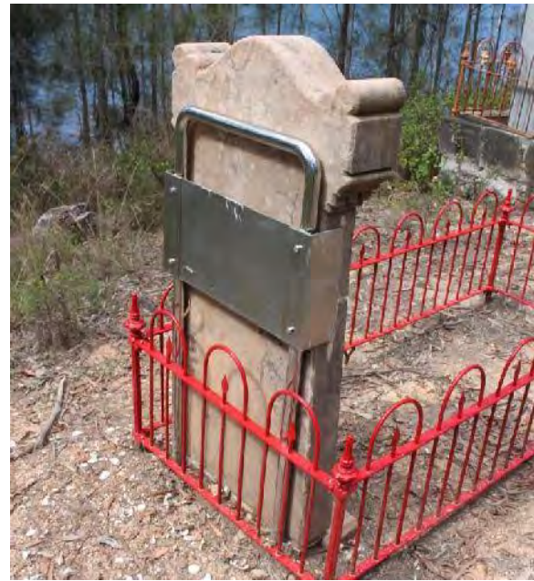
A robust stainless steel frame supports a stainless steel cross-plate and fixing. 2018
