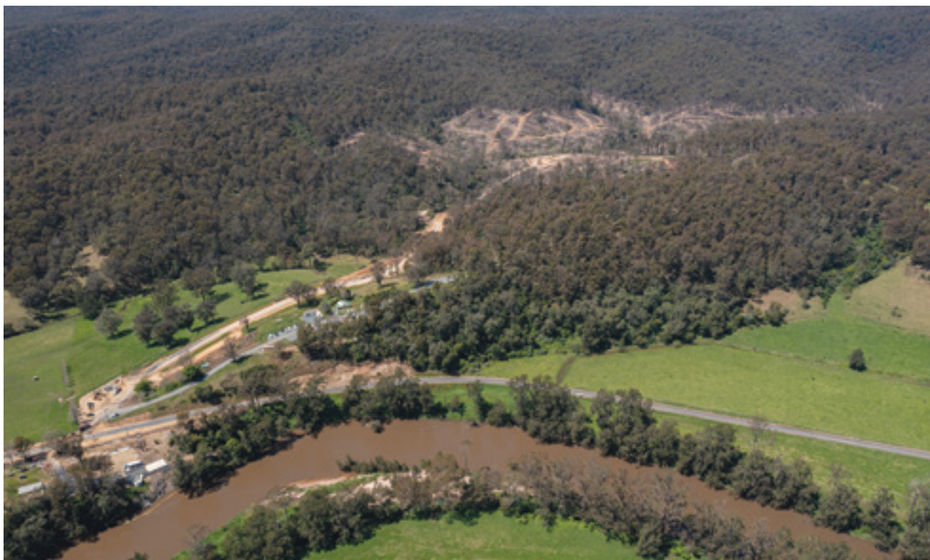
Image: Construction of the new southern dam, west of Bodalla, is on track.
