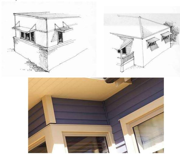
**Eaves.** Properly designed eaves can provide the correct amount of shading and protection for windows and external doors as well as being sympathetic to the coastal aesthetic.
