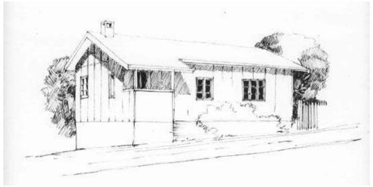
3. Gable roofed cottage with fibre cement flat sheet cladding. Wall lining sheets and cover battens are set out to match window openings. Overhanging gables give some
