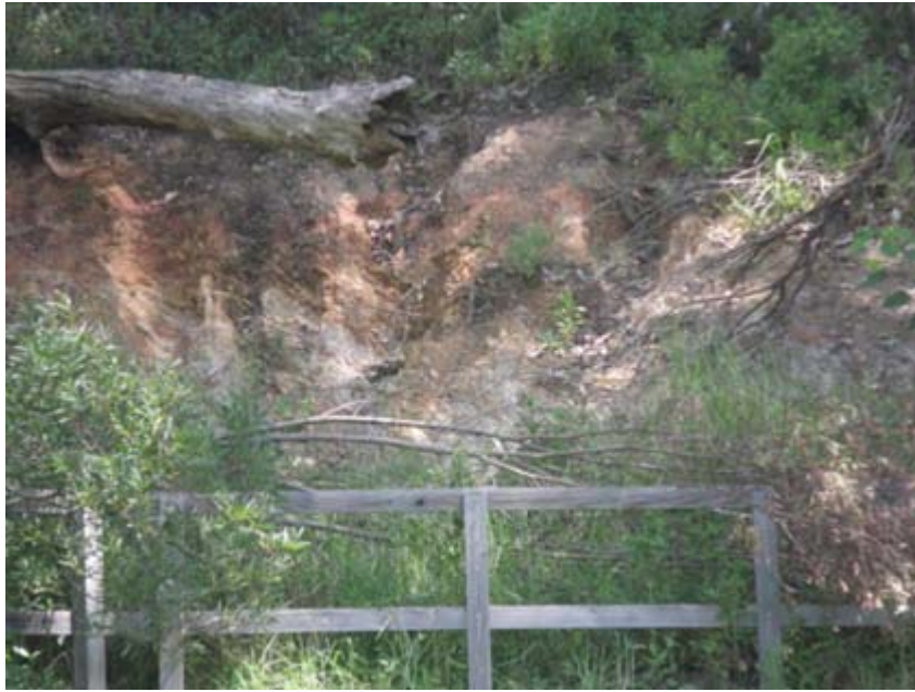
Exposure of weathered coloured clays, southern end of Smyths Oval
