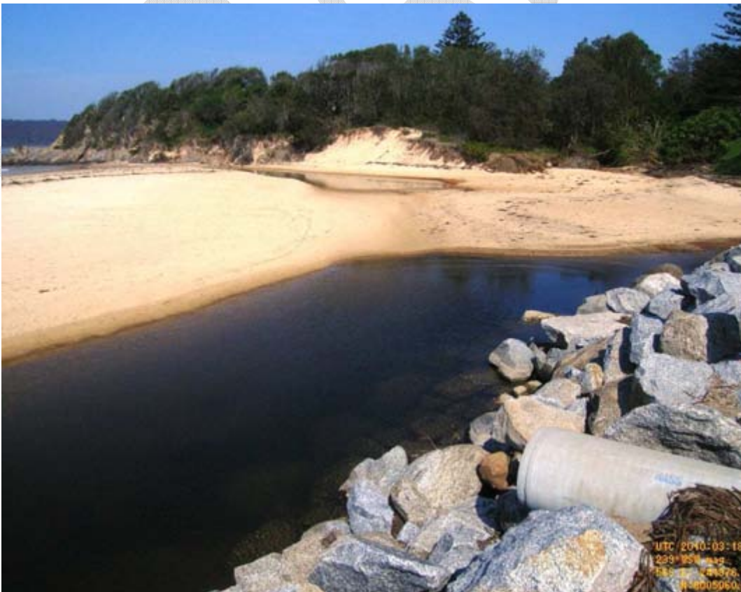
Figure 3.62 – Recent culvert and erosion on dune facing Tuross Beach Holiday Park (March 18 th 2010)
