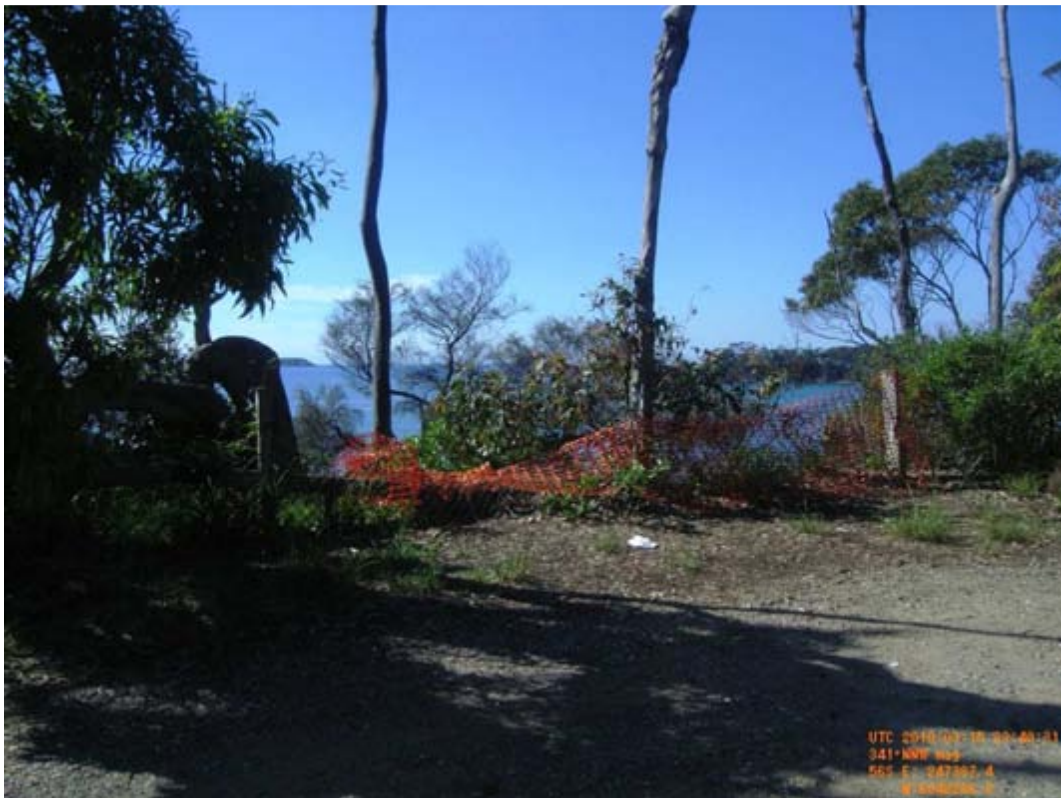
Figure 3.29 – Damaged fencing at the top of the bluff facing Casey Beach (March 16 th 2010)
