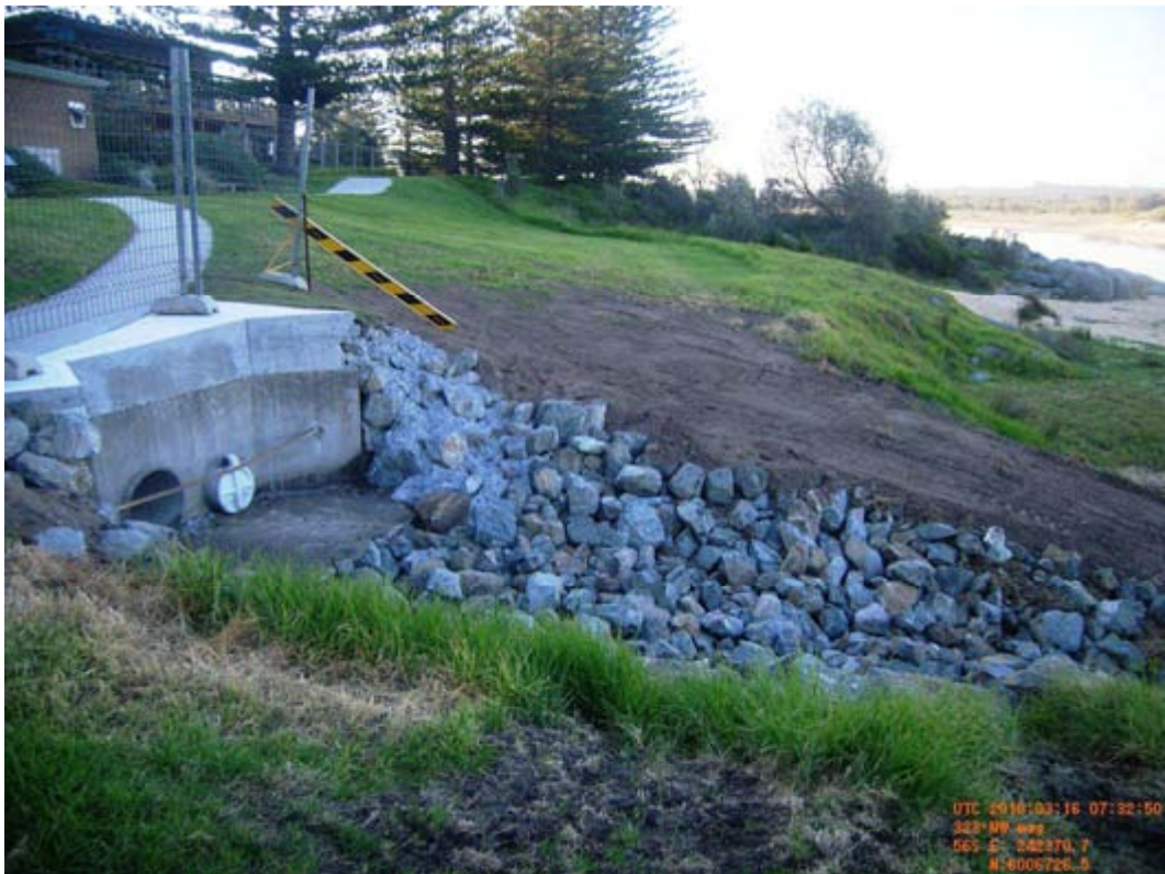
Figure 3.57 – Stormwater outlet under repair at Coila Lake entrance (March 16 th 2010)
