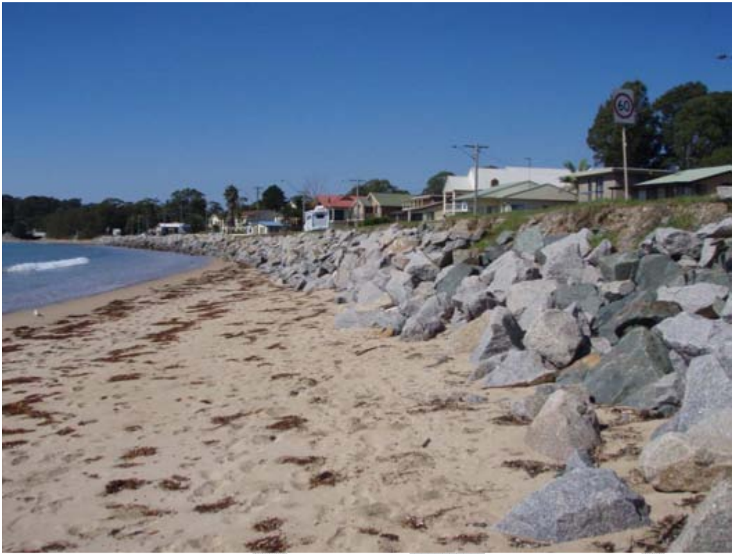
Figure 3.31 – Casey Beach seawall overtopped at northern end (March 16 th 2010)
