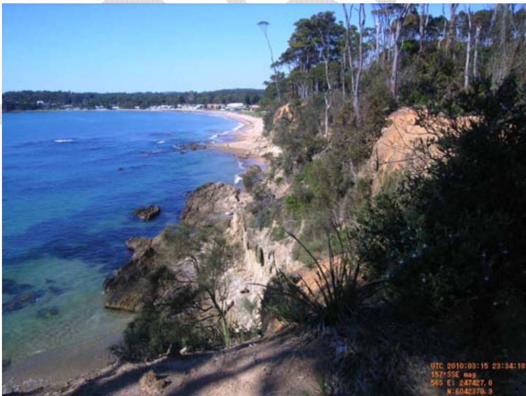
Figure 3.30 – Actively eroding bluff at the lookout facing Casey Beach (March 16 th 2010)
