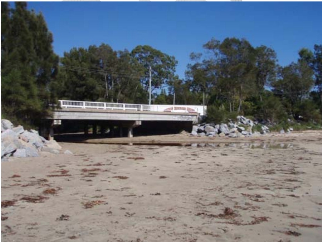
Figure 3.32 – Bridge over Short Beach Creek (March 16 th 2010)
