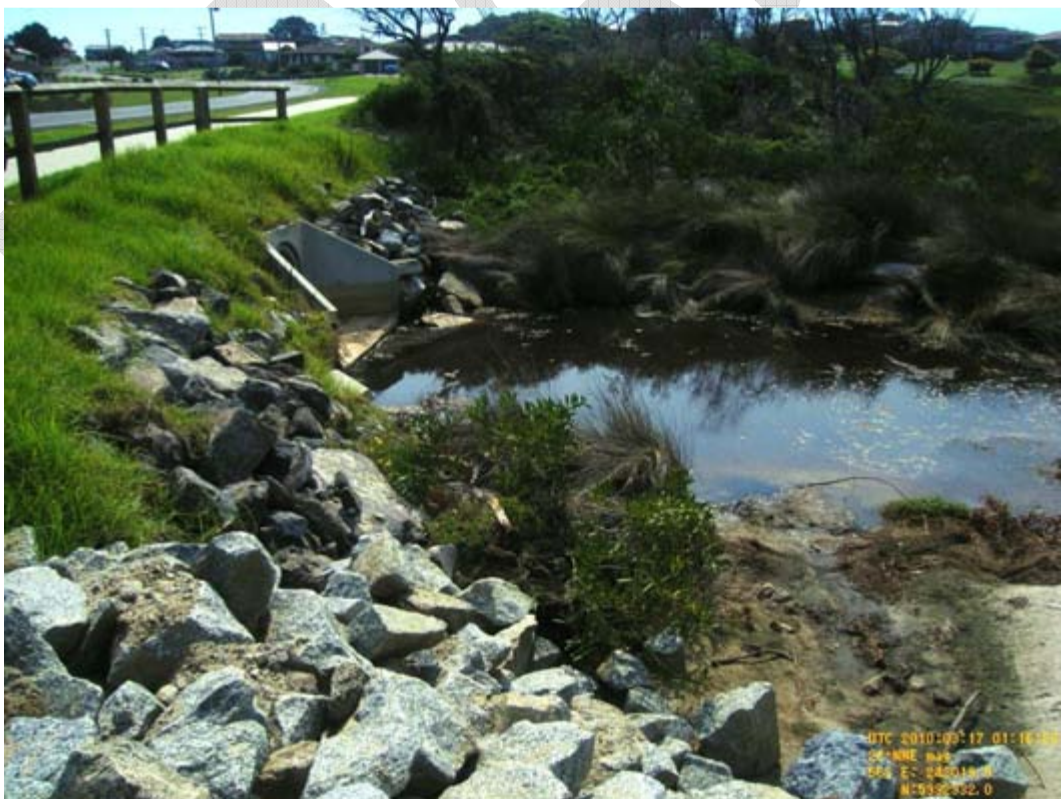
Figure 3.66 – Culvert under Ocean Drive Bridge (March 17 th 2010)
