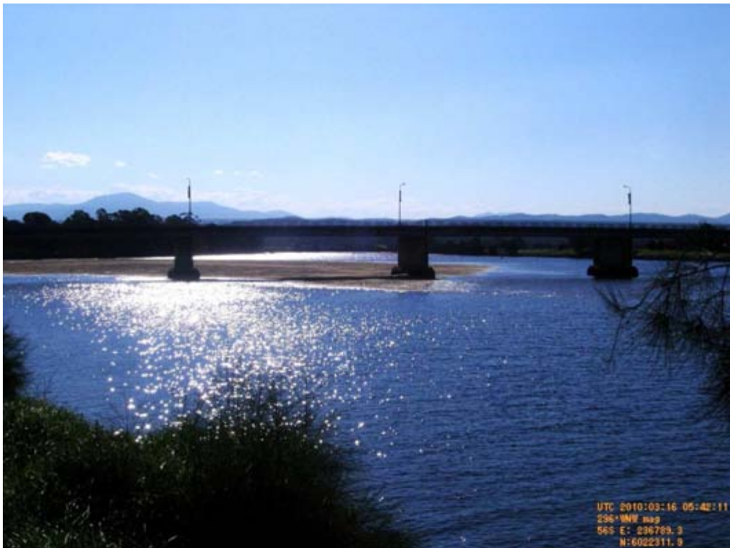
Figure 3.55 – Sand deposition upstream of Princes Highway Bridge along Moruya River (March 16 th 2010)
