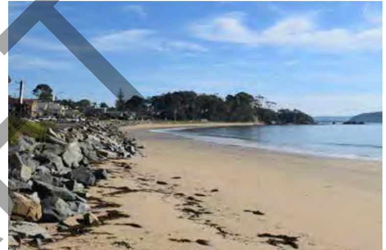
Rock wall along Caseys Beach mitigating coastal erosion
