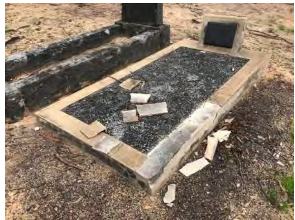
Heat caused the cement render on this serviceman's grave-surround to delaminate. March 2020
