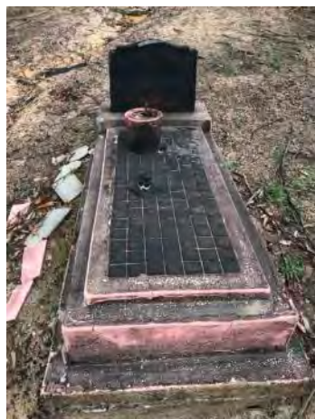
Fire affected monument with heavy smoke damage and defoliation of cement from heat. Photo PGG, 16 /3/2020
