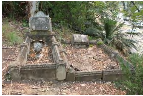
Plot is slipping towards excavated edge 2019
