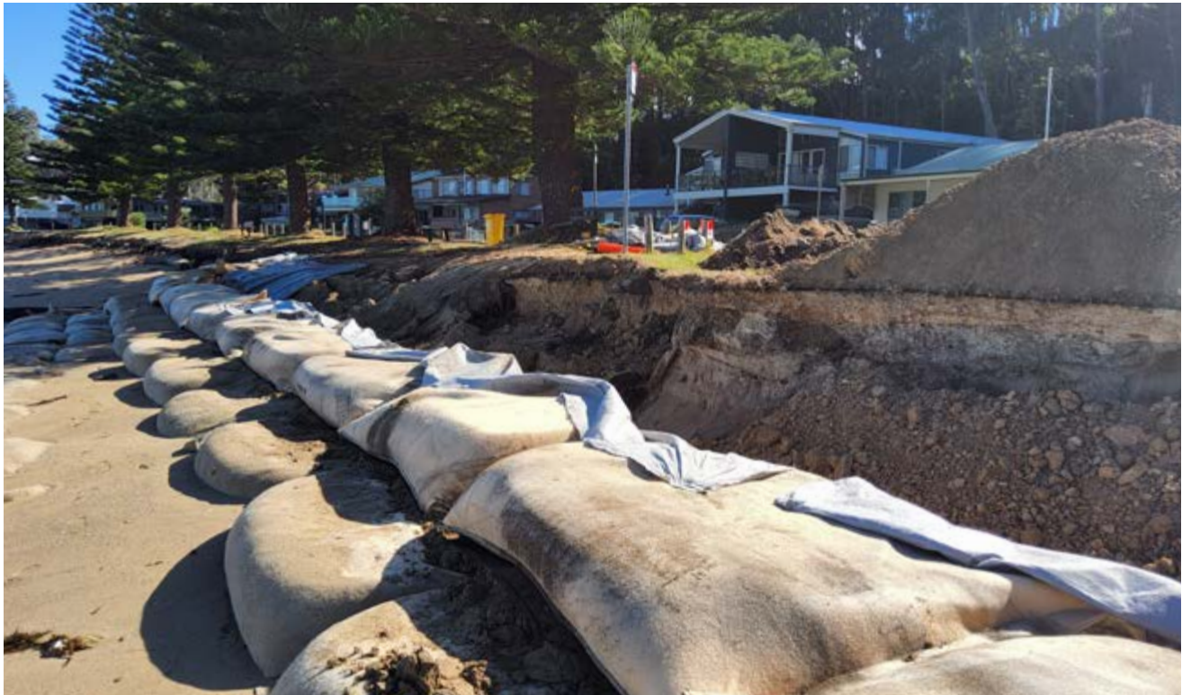
Image: A sandbag structure protects the shoreline at Long Beach, part of the Eurobodalla Open Coastal Management Program
