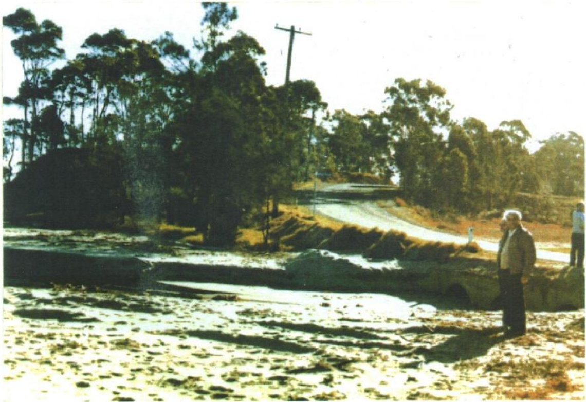
Figure 8-16: Overtopping of Myamba Parade at Surfside Beach (west) 13 August 1986 (NSW PWD, 1989)
