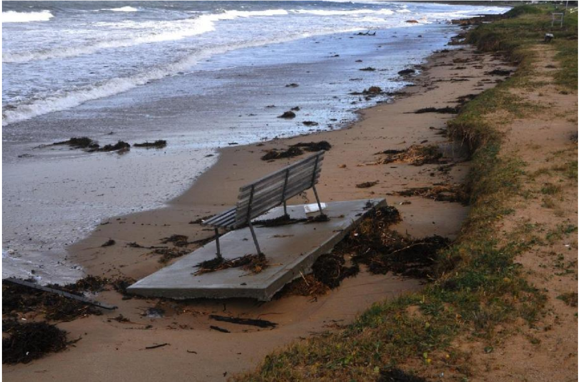
Figure 4-3: Example Storm Erosion, Long Beach, 6 June 2012 (Mr Lindsay Usher)
