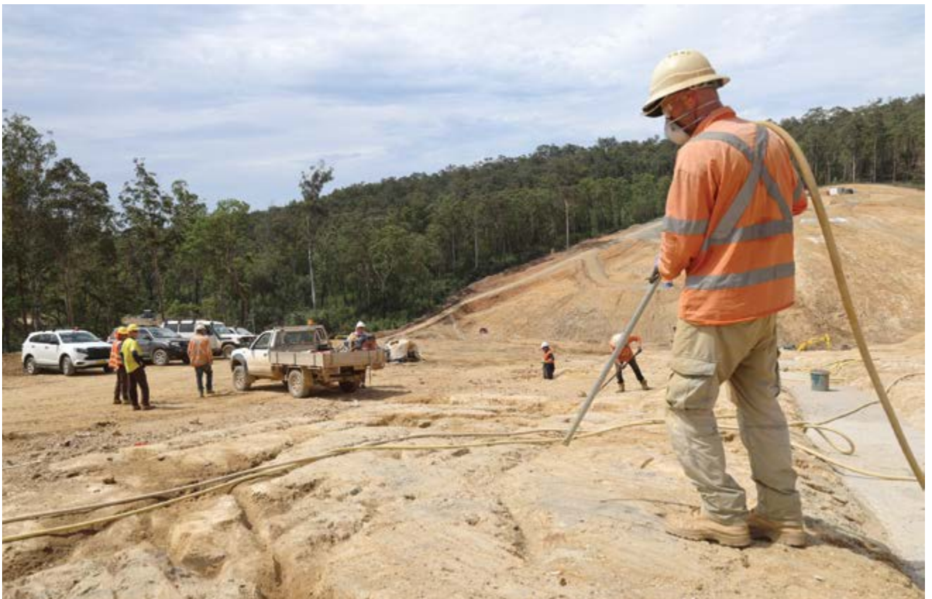
Image: Crews clean out a seam of the new dam wall foundation with high pressure air.
